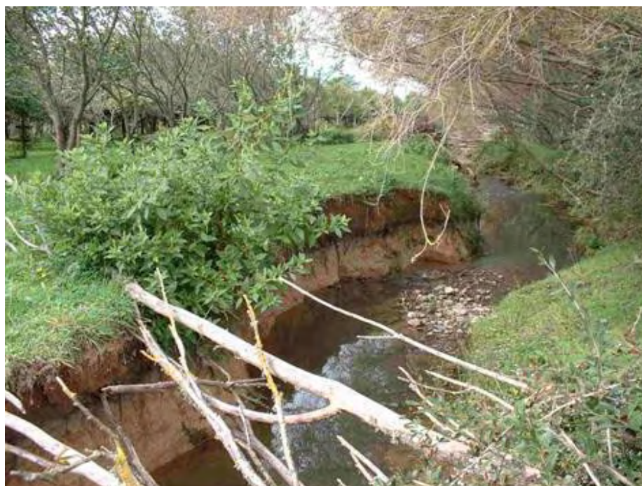
Figure 13: An example of scour erosion; coding and description. Sc (A) o 8 x 1.5 m N: Scour, (active) outside, 8 m long, 1.5 m high, not protected.
