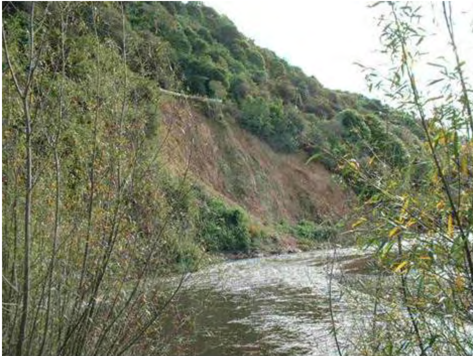
Figure 16: An example of slip erosion; coding and description. SI (A) o ~25 x 15 m V: Slip (active), outside, approximately 25 m long, 15 m high, vegetated.
