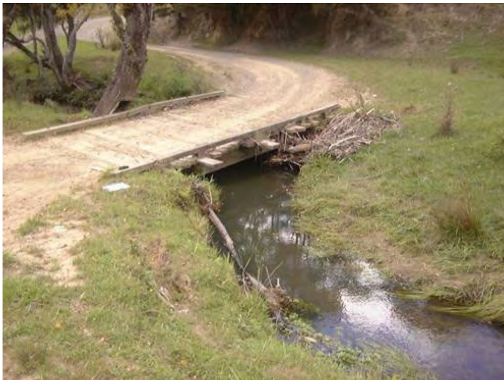
Figure 24: An example of an accessway; coding and description. Bridge: B.
